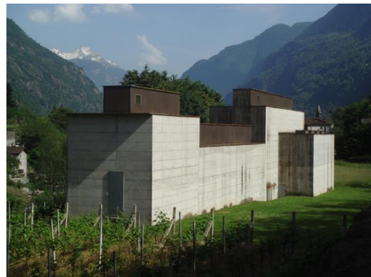
02_MPestalozzi_Transformatorhaeuschen (3072x2304 Pixel)
